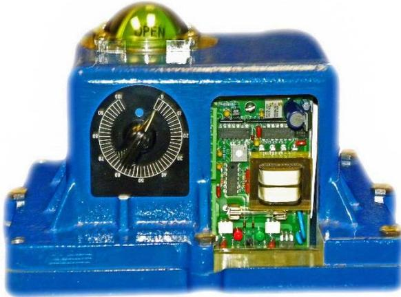
One of the most appealing characteristics of electric rotary actuators is its inherent versatility. Electronic control cards, switches and wiring are easily re-configured to meet the control system needs.
